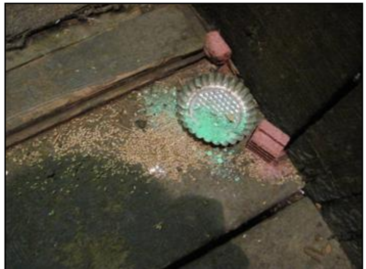
Rodent bait trap utility room 5093
