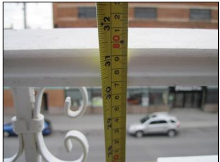
Guardrail's under 32" high
