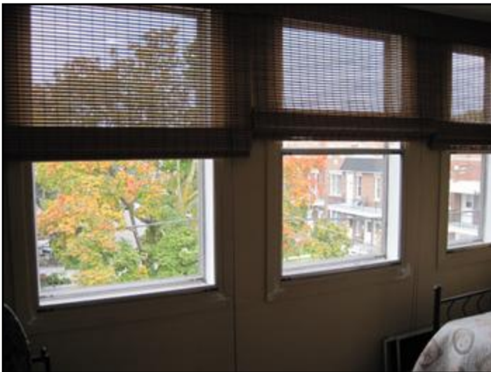
Series of windows sealed with silicone
